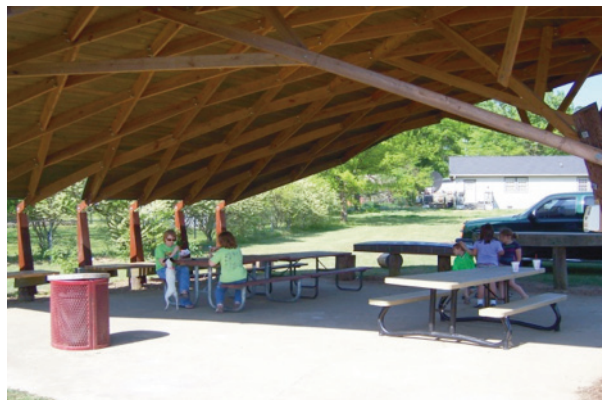
Figure 2. Recreational facilities utilizing preservative-treated wood. Top, a ramp for scaling a bluff at a state park. Bottom, a city park pavilion.
