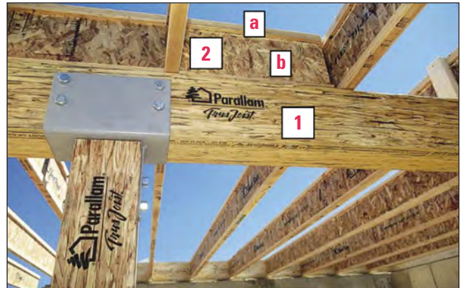
Figure 5. A construction site using wood composite products. (1) Parallel strand lumber. (2) A wood I-joist consisting of (a) laminated veneer lumber and (b) oriented strand board.
