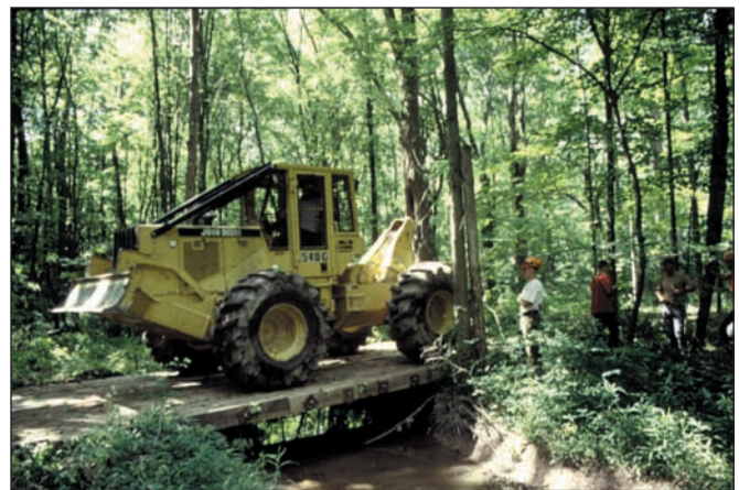
A portable logging bridge provides easy access to the forest on both sides of the stream.
