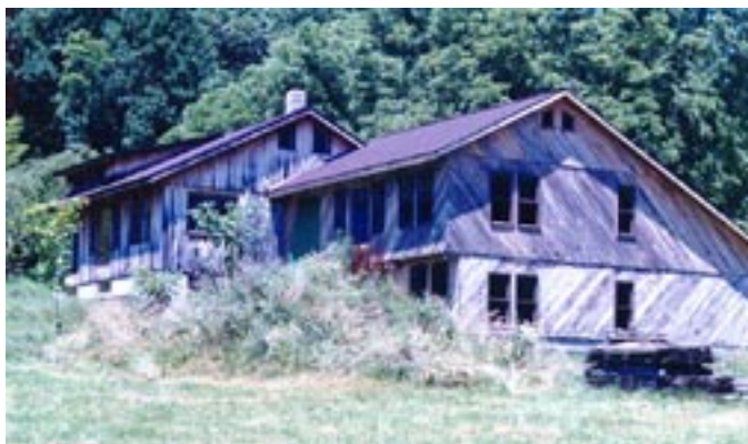
Home built using yellow poplar lumber milled on a portable sawmill from trees grown on a farm in southern Ohio.
